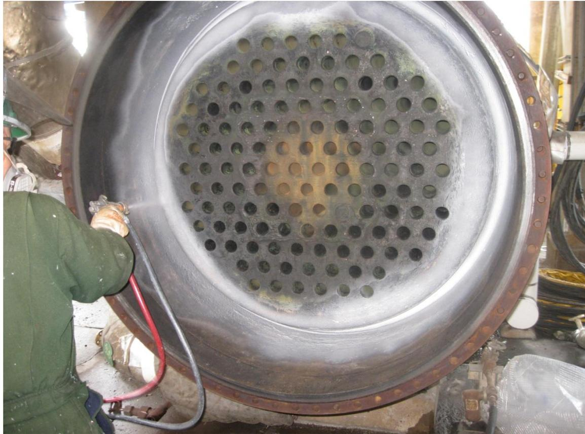
Application (spraying) of first coat of EZ De-Coke to TLE inlet tubesheet surface.
