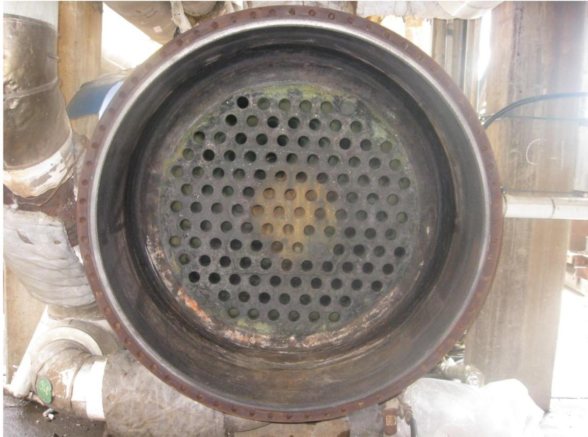
Hydro-blasted, dried and hand-brushed TLE inlet tubesheet surface ready for re-coating.
