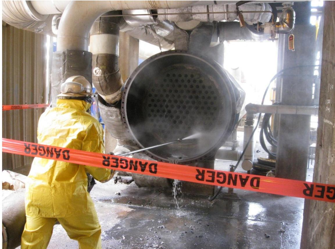
Hydro-blast cleaning of TLE inlet tubesheet surface. No Chiseling.
